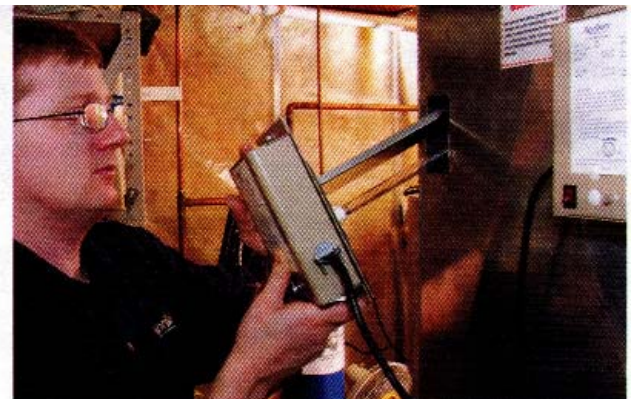
To continue the work preceding a successful UV lamp installation, make sure the unit base can be placed through the rectangular opening in the duct.
